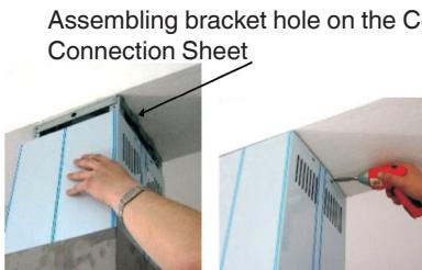
Assembling bracket hole on the Ceiling Connection Sheet
